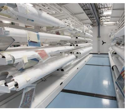
Large Viking by Spacesaver cabinets were fitted with shallow drawers to maximize vertical space within the cabinets, and the cabinets were mounted on carriages and rails to eliminate wasted space in the aisles. The cabinets hold a variety of smaller artifacts, from historic dishware to medals and belt buckles.
